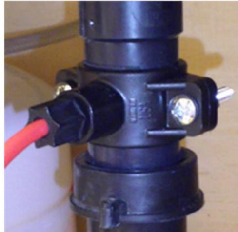
Fig. 5 Drain saddle
